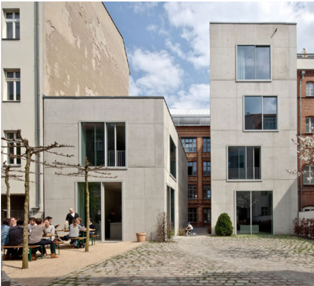
CHIPPERFIELD - COURTYARD CANTEEN - BERLIN
