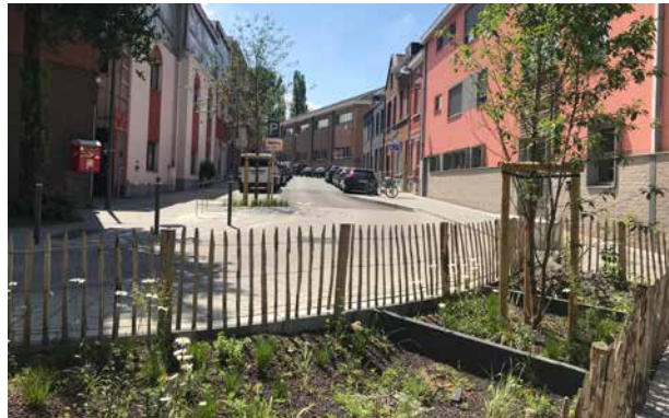
↑ A water basin separates the road from the pavement and collects run-off water on Rue Essegheem in Jette. © Suède36
